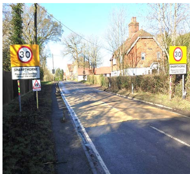
Photograph 2 – Existing 2015 Traffic Calming 'Gateway'
