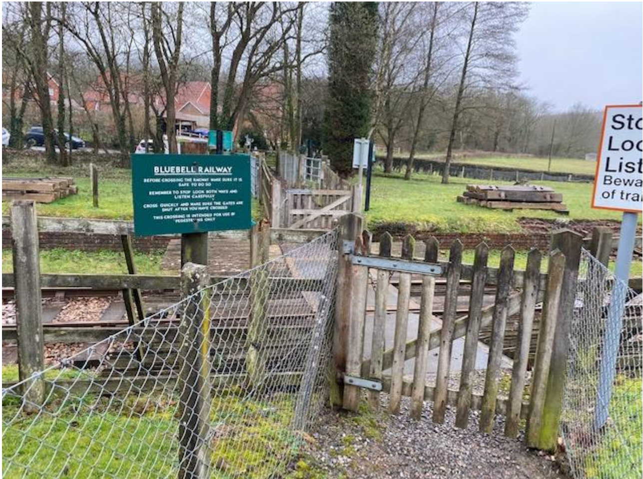
Figure 4-7: Railway At Grade Crossing Site Visit Photo
