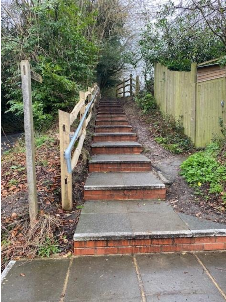
Figure 4-9: Footpath Entrance Site Visit Photo`12
